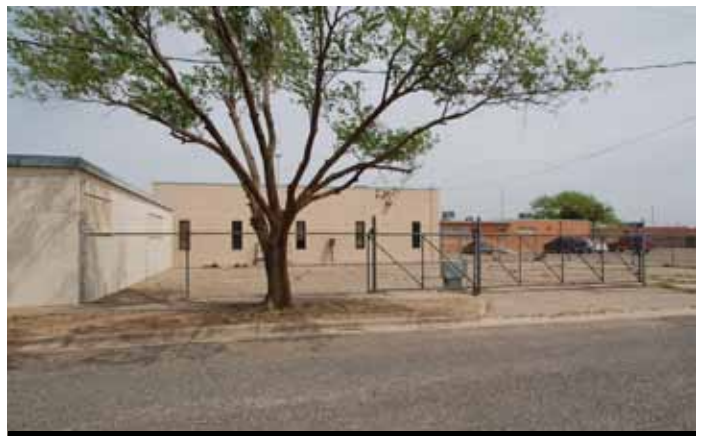
Workshop 1,500 SF & Stack Yard
